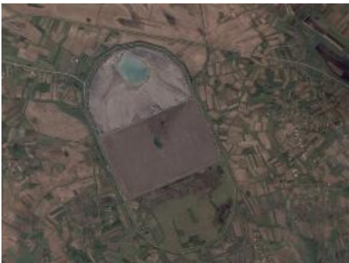
Figure 104 Orthophoto image of the ash landfill near Obrenovac
